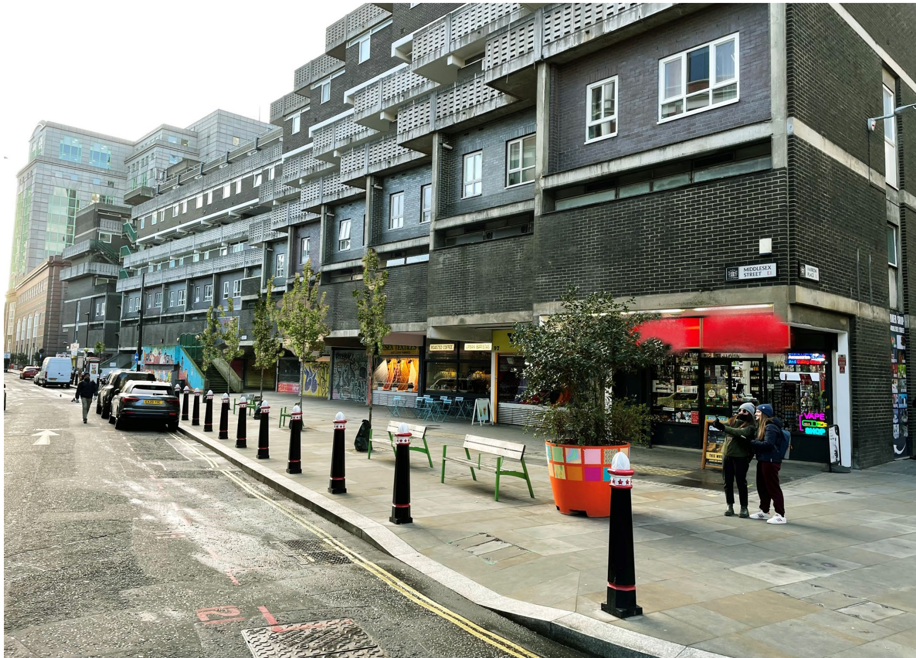
Middlesex Street central area – street trees and seating replaced the concrete planters, creating more space for people walking and wheeling and opportunities to rest. The function of the street remains unchanged.
